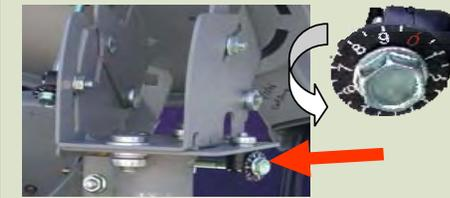
**(10)** Tighten down the Azimuth bolts and verify signal via the IRD
